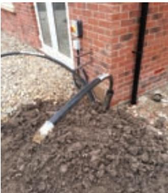
**Gaining ground:** Kensa has pioneered a novel system architecture with individual heat pumps being served by a communal ground array. Photo shows borehole pipes to connect to the unit
