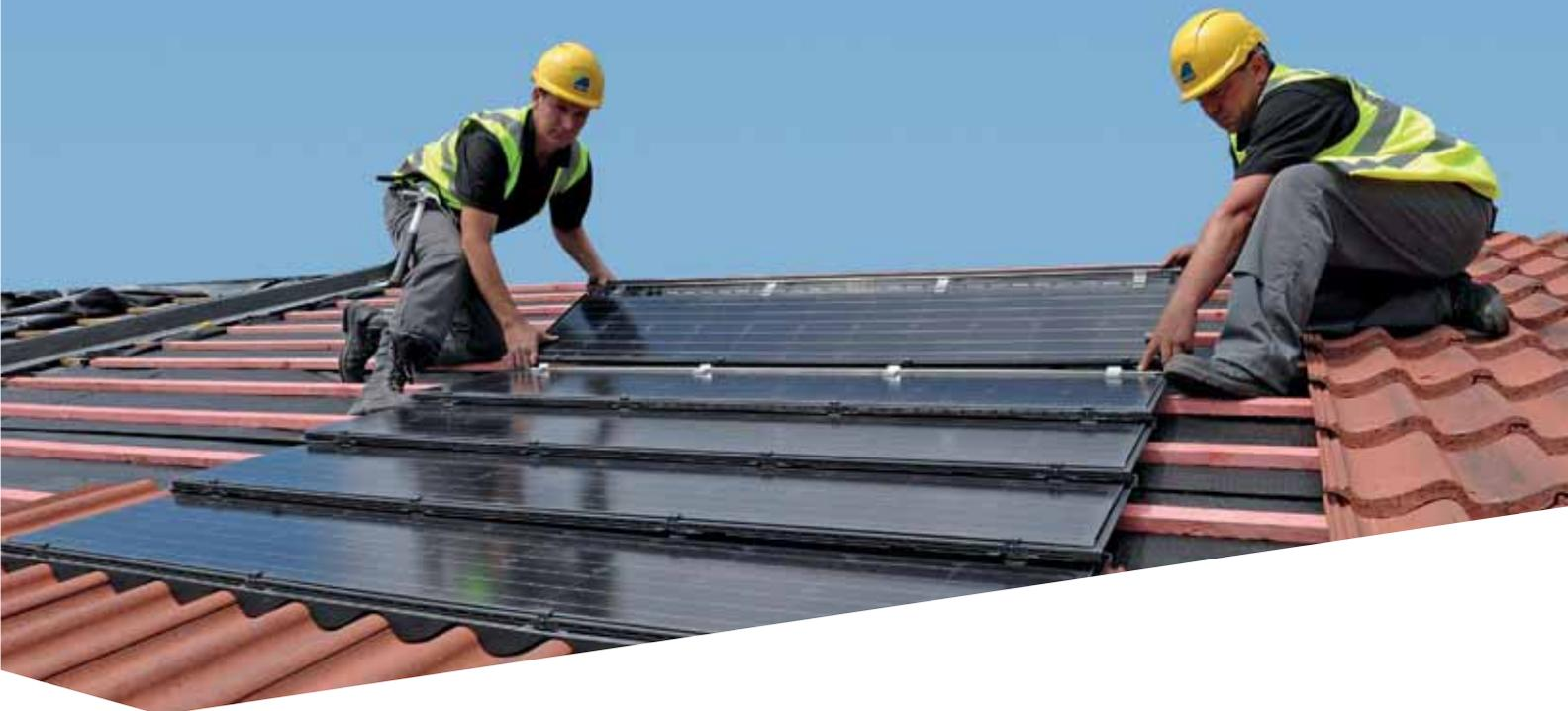
Fully integrated, our Solar PV tiles are easy on the eye, easy to install and are guaranteed weathertight with our 15-year Roof System Guarantee. They're compatible with eight of Redland's most popular tile ranges, including slate, profile and plain.
